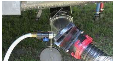
Clean-Out Hook Ups
