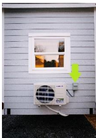
Mini Split Main Shut Off/Disconnect
